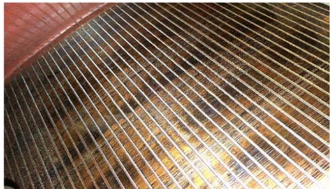
Figure 8: Threading caused by excessive humidity, contaminants, and/or low spring tension
